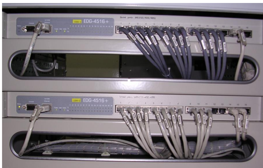
Figura 13 - Conversor EDG-4516+, RS232 / Ethernet.
